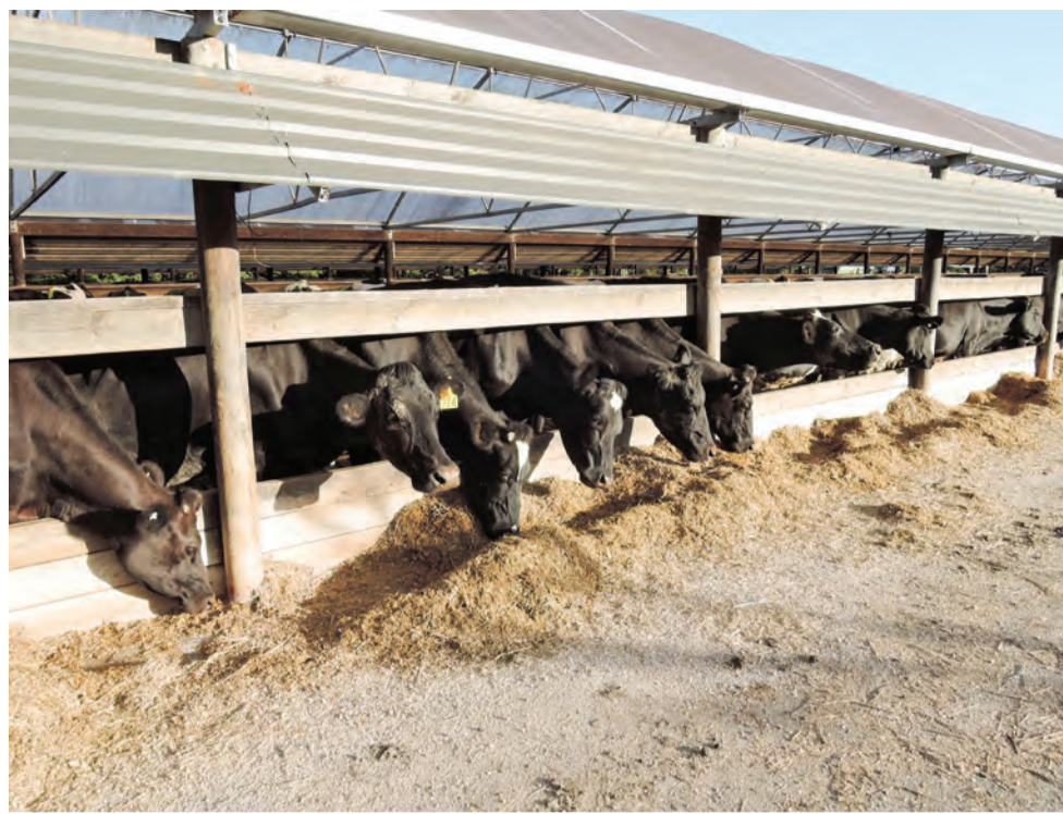
Investing in a slatted floor barn can have benefits if done right.
