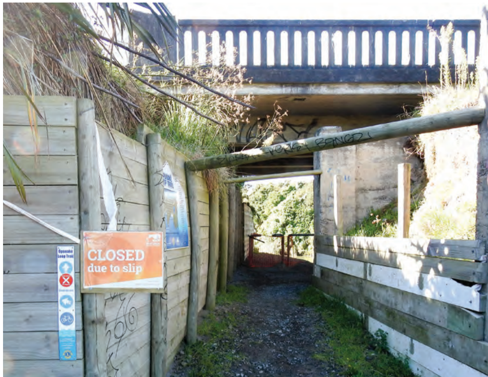
Part of the Opunake Loop Trail remains closed while repair work takes place.
