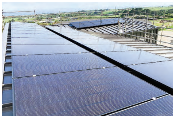
Oakura Water Treatment Plant solar panels.
