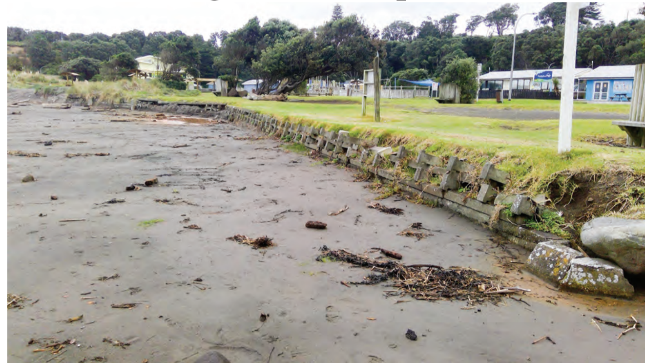
The Opunake Beach retaining wall is being replaced.
